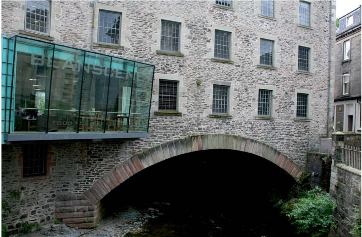
Rock is exposed in the river bed so foundations were clearly not a problem. This skewed face has nicely dressed voussoirs of uneven thickness, with some thinner voussoirs near the springing.
