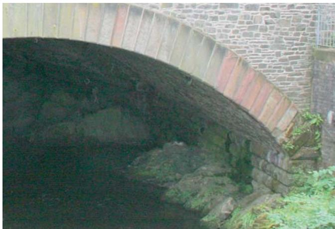
Cropping this picture and pushing the light severely reveals a kink a few metres upstream of the arch face. The remainder of the structure is essentially square. This skew arch constructed from random rubble surely gives the lie to the idea that bedding of the stone or brick is structurally significant in skew bridges.
