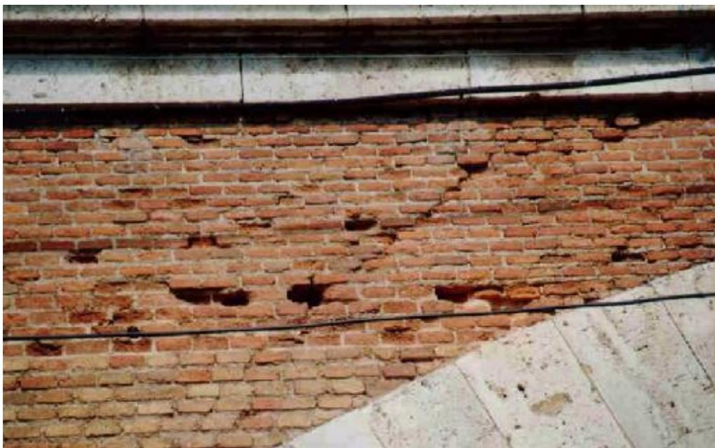
This, yet closer look is obviously a different span. The line at which the weathering starts is very clear. There appears to be a diagonal crack in the brickwork but it might just be a construction joint, perhaps where the skilled bricklayers worked away from the ring and produced an easy edge for the improvers to work from.
