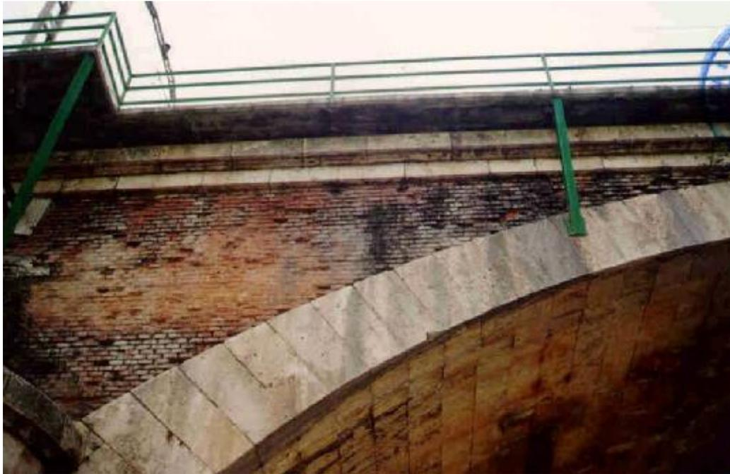
A closer look shows more of the nature of the weathering of the brick. It also shows clearly that the expressed ring (at least) is tapered, beautifully fitted and has tight joints.
