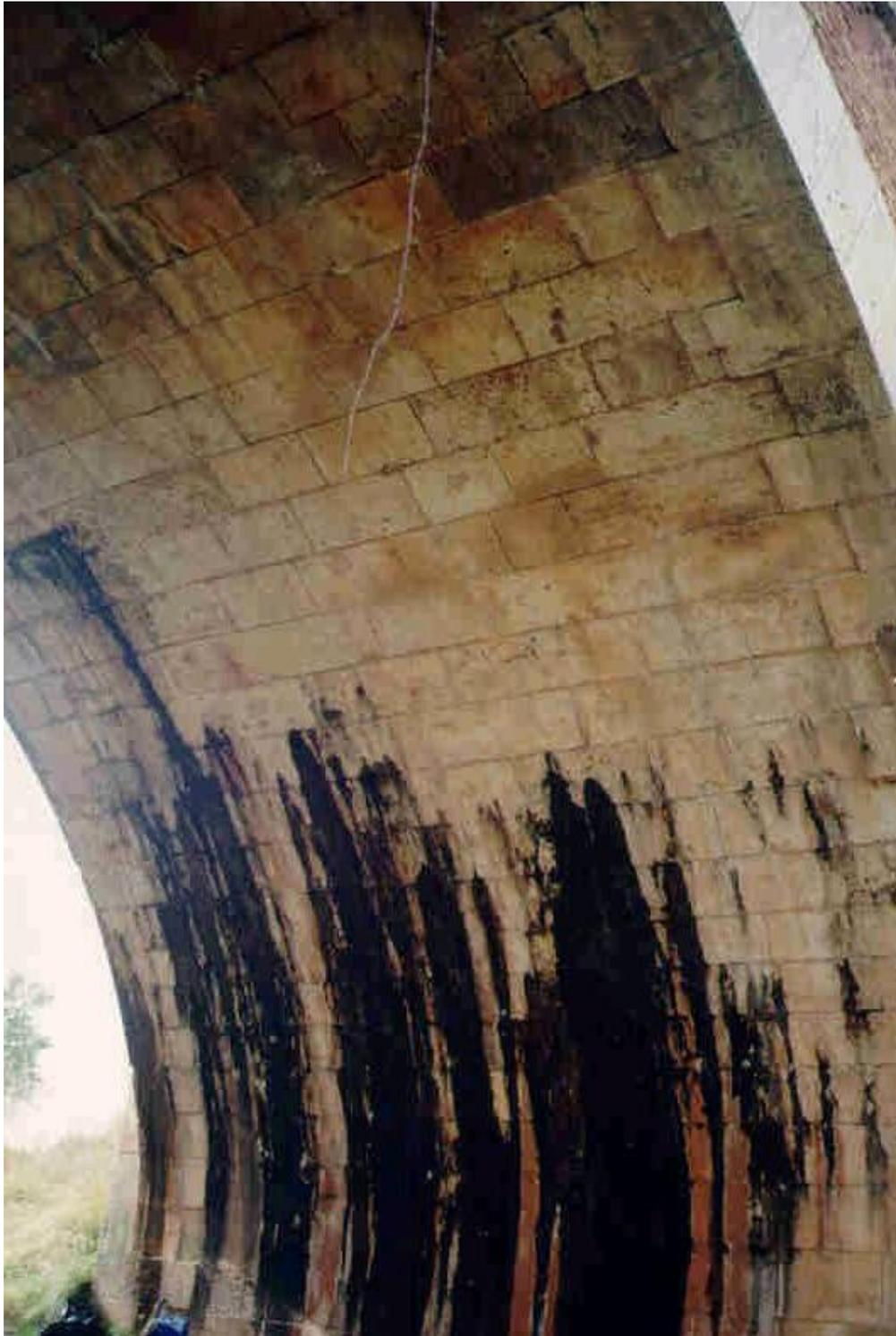
Look underneath the arch and there are pronounced water runs from well up the curve. Notice, however, the highest one at top left which is obviously of a different set. That isn't a crack but a bit of vegetation hanging down.
