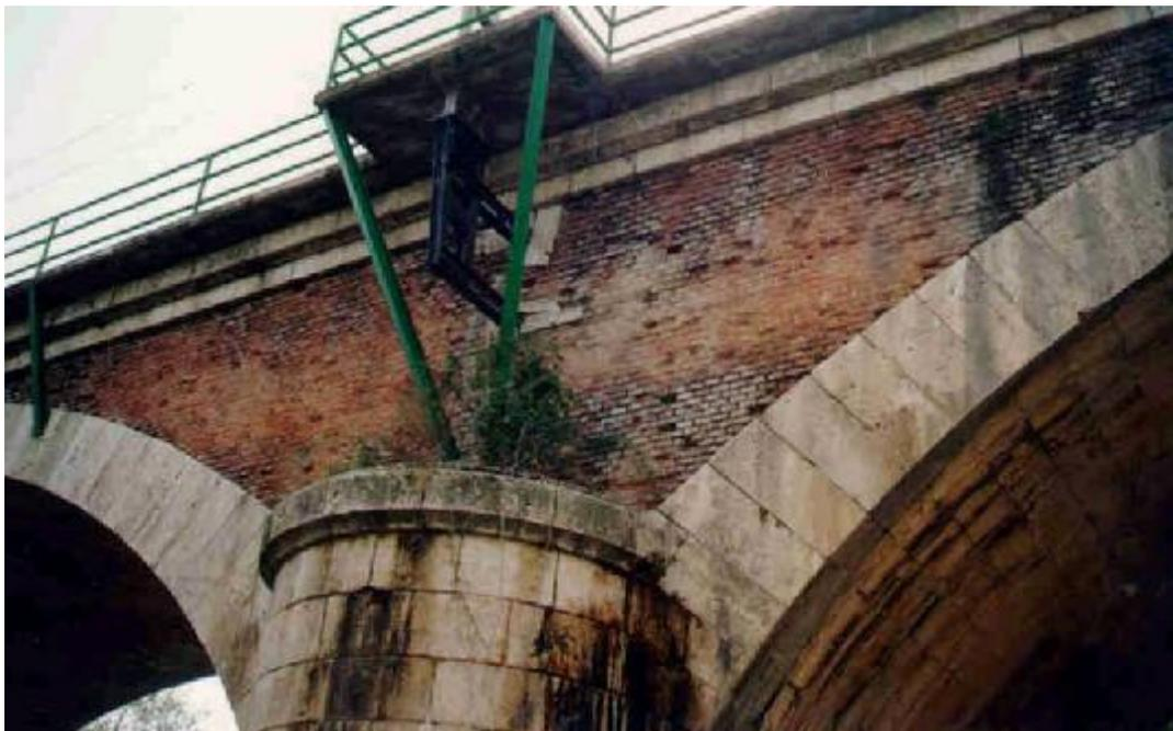
A look at the spandrel wall shows a band of weathering in the brickwork. Look carefully at the bottom right and you will see that the bottom edge of this corresponds with the lower layer of water runs in the soffit. Look back to the first picture and the correspondence of the water runs and the weathering levels in the brick becomes obvious.
