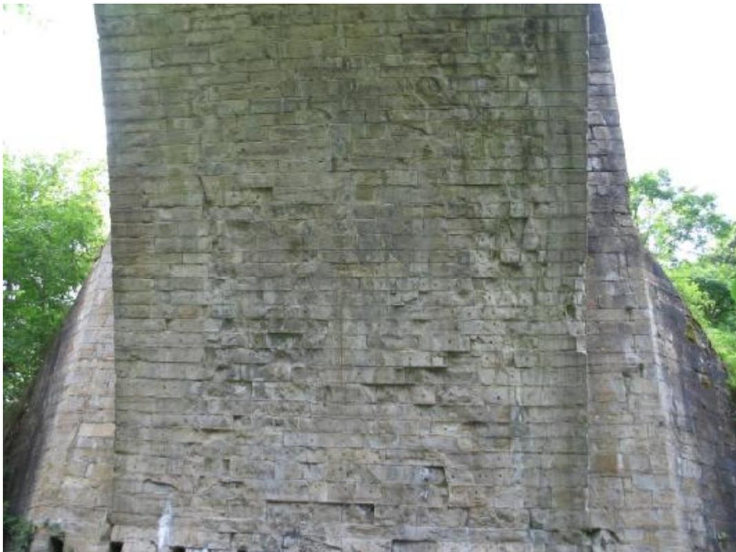
The damage extends upwards for some distance and then largely stops. There is similar damage near the arch crown and at the opposite springing.
