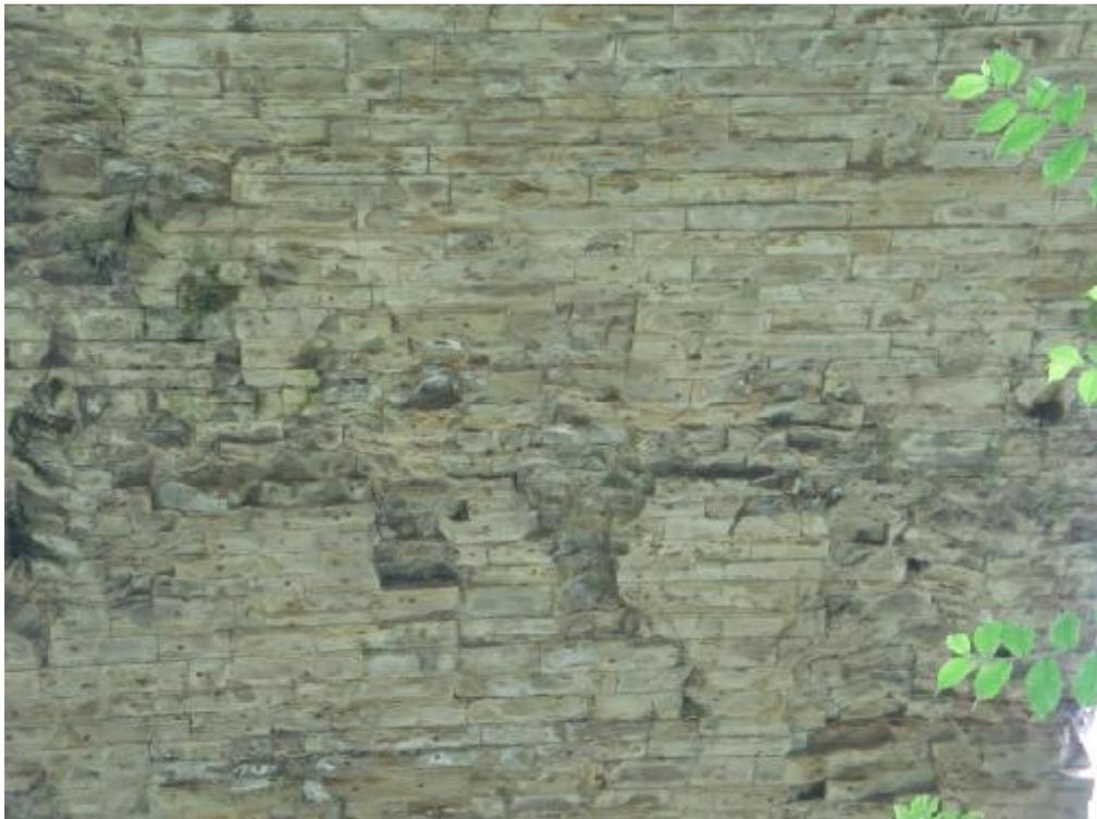
With a span of 30m and semi-circular form. The spandrel walls are about 17m high. To contain earth at such a depth they would need to be very thick, much thicker than the width of the bridge so the bridge would end up being solid masonry. That must be regarded as unlikely possibility.
