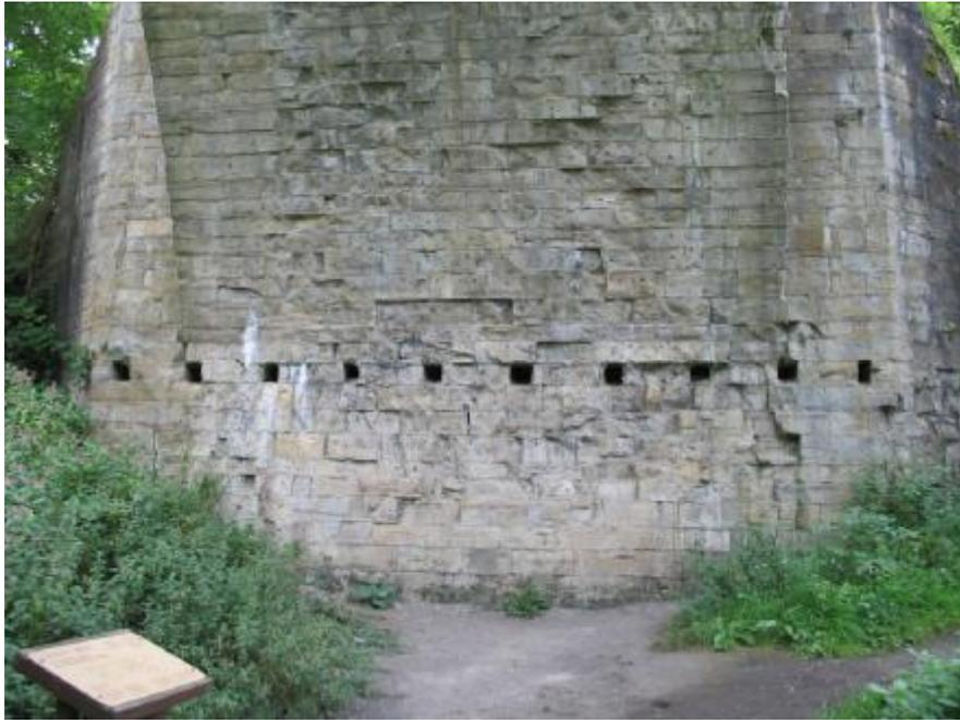
This picture also shows severe deterioration of the stone, which is, interestingly, concentrated beneath the arch and more or less absent at the edges.
