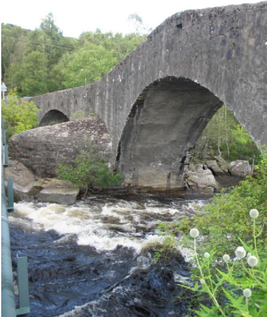
Here we see the “double arch” referred to in the contract. The gunited soffit is not a happy thing. It is most likely done as a cheap alternative to pointing but the harm it does is untold. It also obscures the nature of construction of the arch itself, though the selected slate like stones exposed on the face are quite likely to have been used through the full width.
