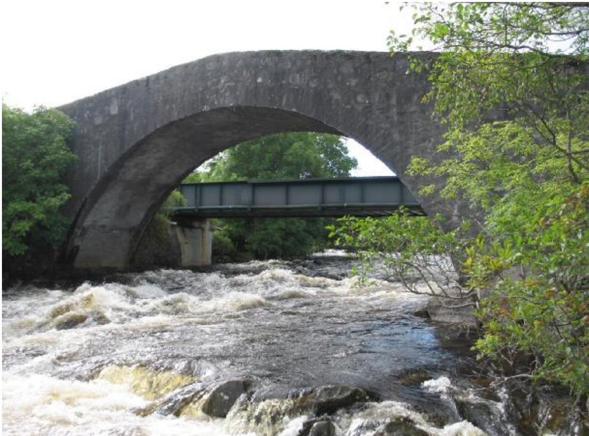
The good condition in which the bridge is found is probably a result of the replacement built in the 1930s to carry heavy machinery to the nearby hydro power station. This picture was taken in summer and the river doesn't look at all friendly to the building of a timber centre for such a large span. It would be wonderful to know more of how it was built. We are entering the era of the Civil Engineer by this time. John Smeaton was born in 1724, James Brindley in 1716.
