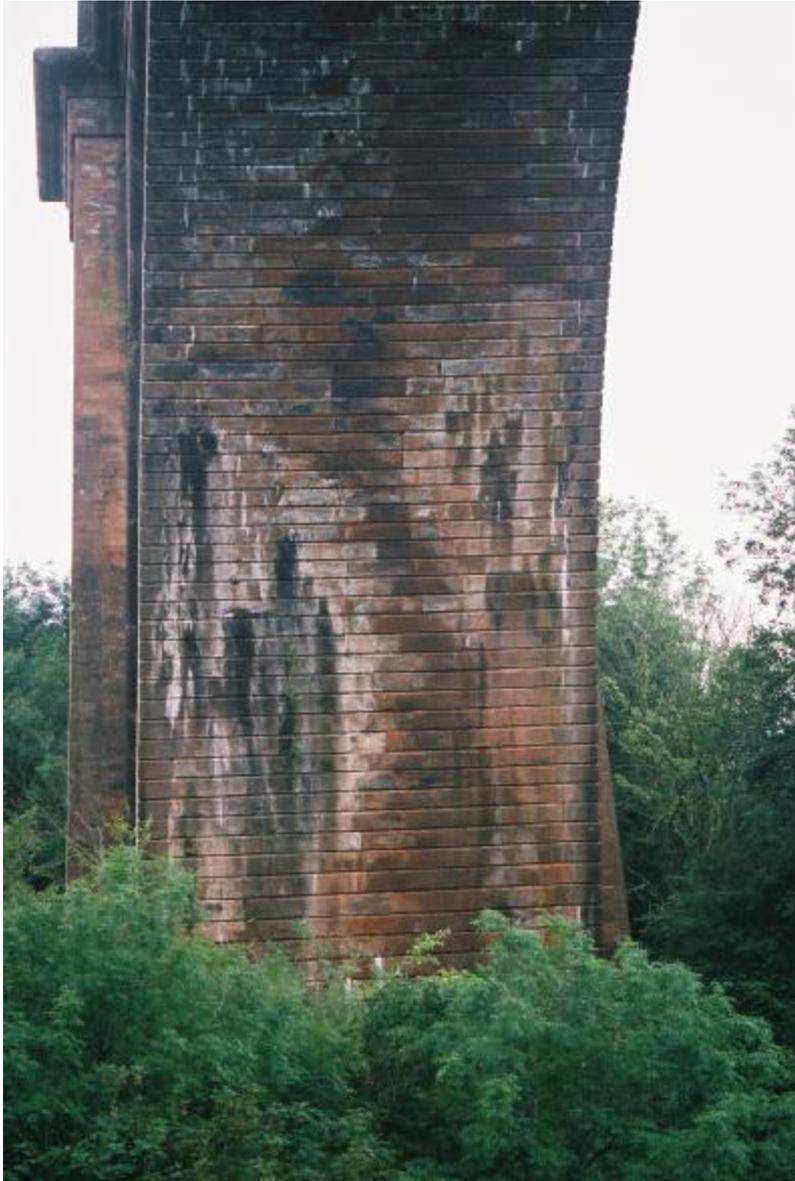
This picture shows about half the arch. The water stains show the top of the solid masonry. The bridge is of hollow construction with internal spandrel walls under the rails capped with stone slabs. There are also cross walls providing support and these show in the staining on the elevation on page 1.
