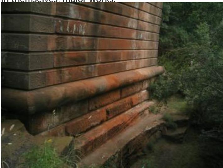
The scale of the stonework is seen from this closeup of the abutment. These Voussoirs are about 0.5m thick and some are nearly 2m square. Lifting them the 60m from the river with the hand winch on the Gantry crane must have been a serious undertaking.
