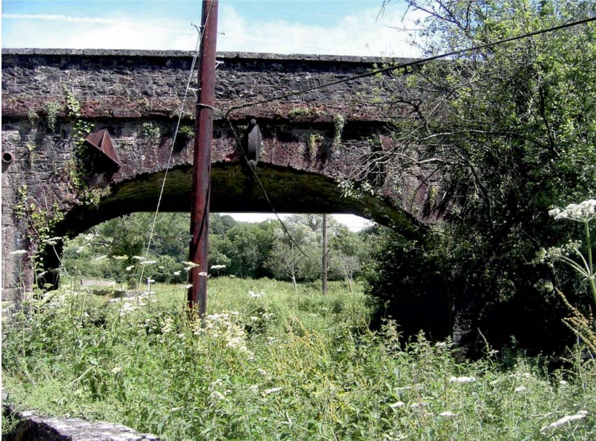
This picture was taken deliberately from a point at which the faces of the piers are not visible . The river goes to the right of the right hand pier and the road to the left of the left pier. The arch spans about 25ft on the west side and 35ft on the east. That's 7.6 and 10.7m.
