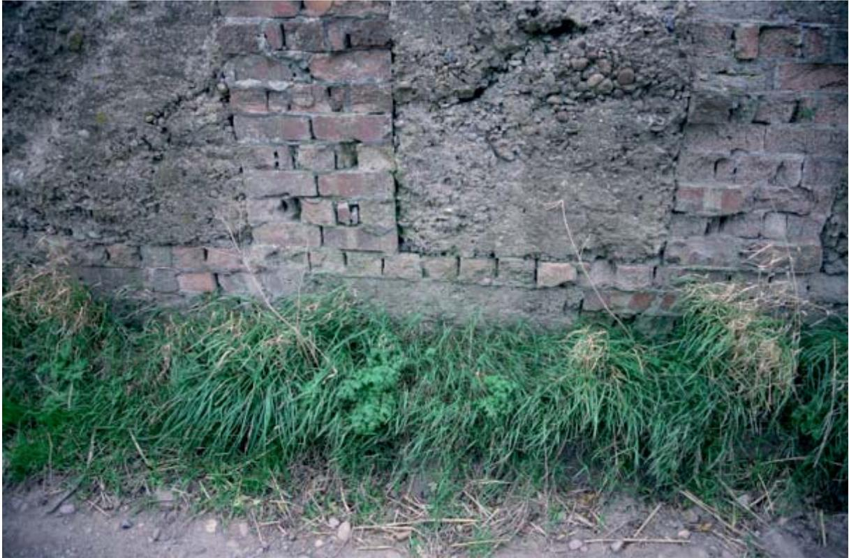
A close up of the cut face shows relatively low quality concrete and even the brickwork has mostly empty perpenders.
