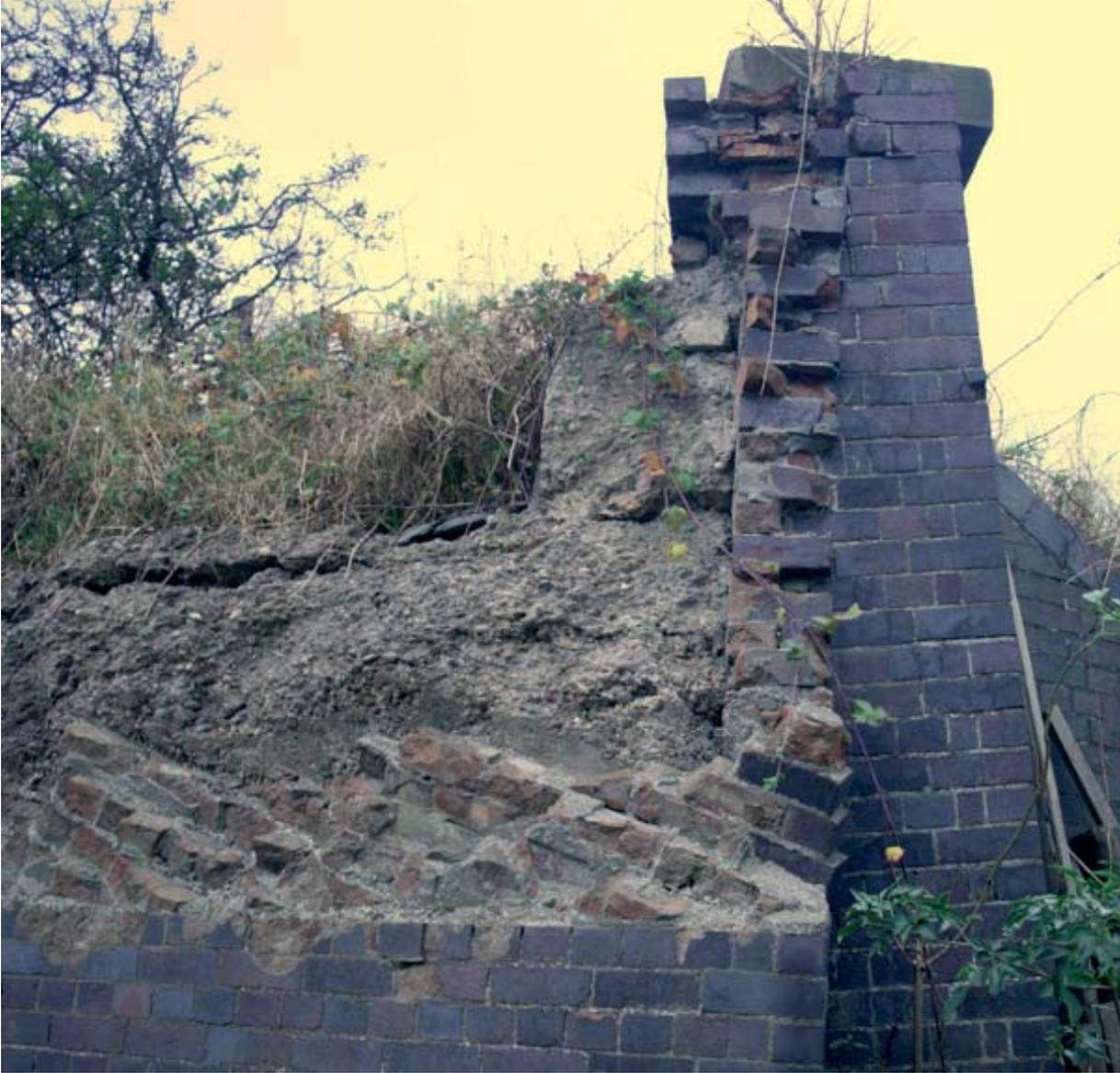
Here we can see an array of detail. Not only is the relatively thin arch backed with concrete, but the spandrel wall is built a mere 9" (225mm) thick and then concrete cast against the inside.
