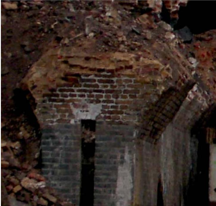
This final segment of the picture shows where the pier was pierced with a cross vault. Looking at the construction here the vault almost certainly didn't rise as far as the main arch but it did divide the arch considerably and induce a substantial additional stress in the pier.
