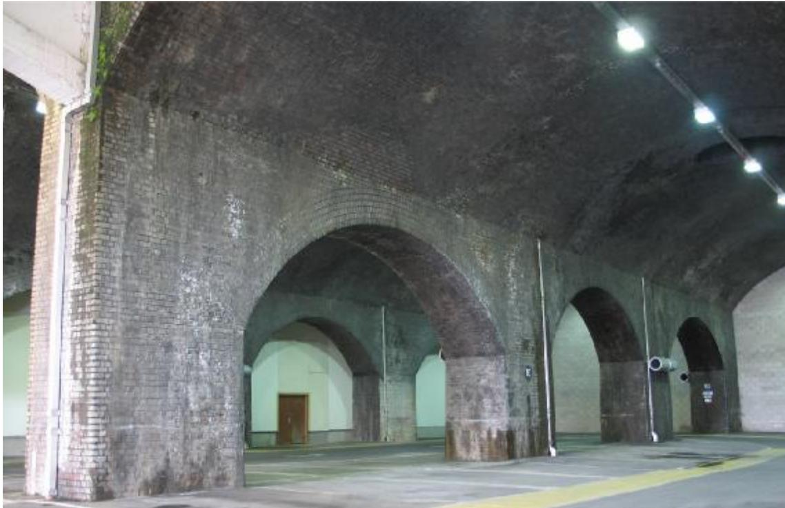
The inner arches in the piers are different. 27ft span instead of 30ft. Note the oval void at the crown of the main arch. These were light wells in the old dispensation.
