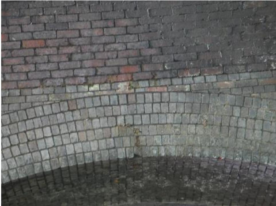
A closer look shows the crack penetrating perhaps three courses. Remember, though, that the arching action is not constrained to stay within the brick rings.
