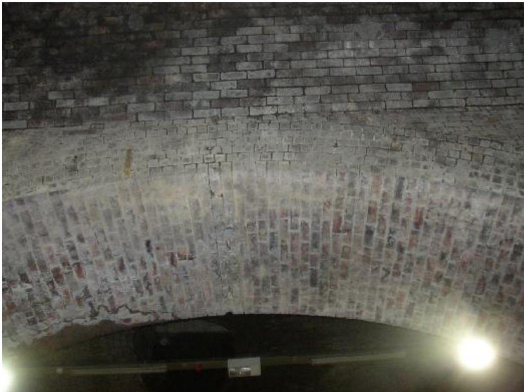
The natural spread of the arch on decentring creates an upward shift in thrust at the crown and in this case, a slight spread and crack at the intrados.
