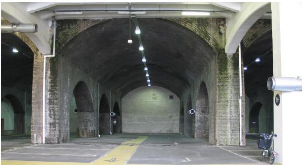
The concrete beams support a new carpark. The piers taper as is visible here.
