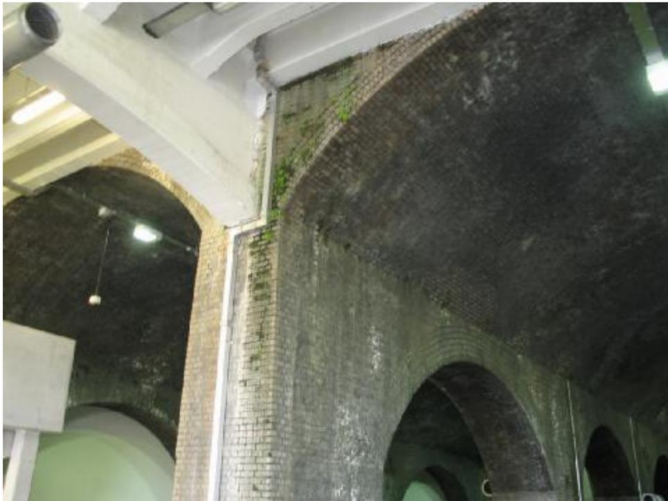
Interesting that rounded corner bricks were used at working level but hard square corners above.
