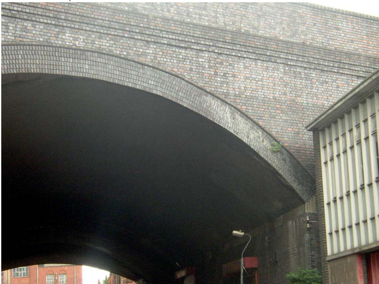
The arch itself is of blue brick, as is the rest of the viaduct. To the left of the picture is the undercroft of Moor Street station. Now a car park, it was originally a goods shed with lifts to move goods wagons up and down to the railway and traversers to carry them at right angles from track to track in the shed. To the right, the viaduct becomes progressively narrower.
