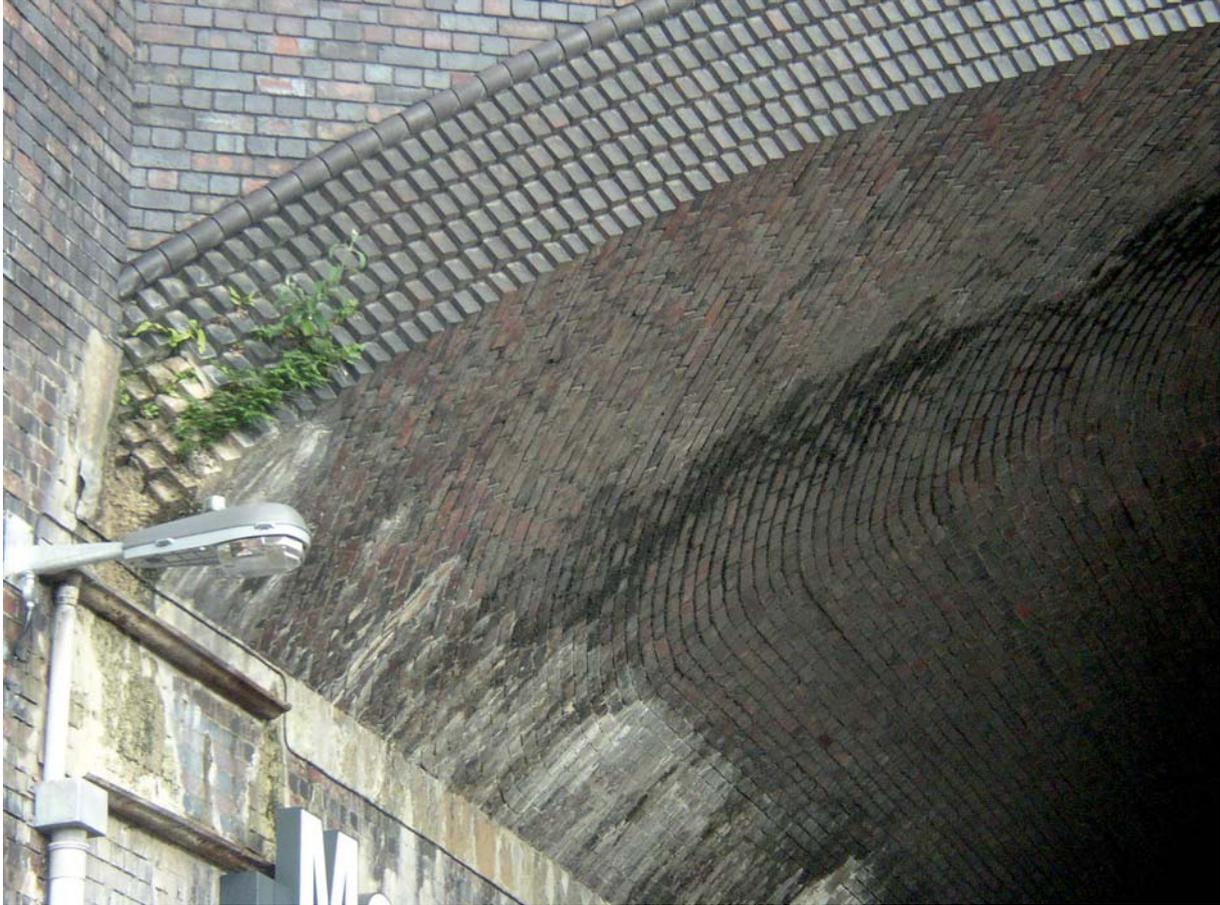
The picture above shows the nature of the arch construction. The skew angle on this face (zoom in on the map to see) is about 40 degrees. At the other face there is a much smaller skew in the other direction. The skew edges are accomplished by sweeping the brickwork round a curve so it runs parallel to the abutment over most of the width but still meets the skew edge more or less at right angles.
