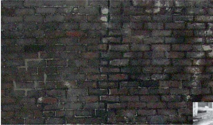
One good reason for bringing the courses back to parallel away from the edge is that it allows construction joints to be made. The bricklayers were very good at fitting in the bricks on these joints but they remain visible if you look for them as you can see at the left.
