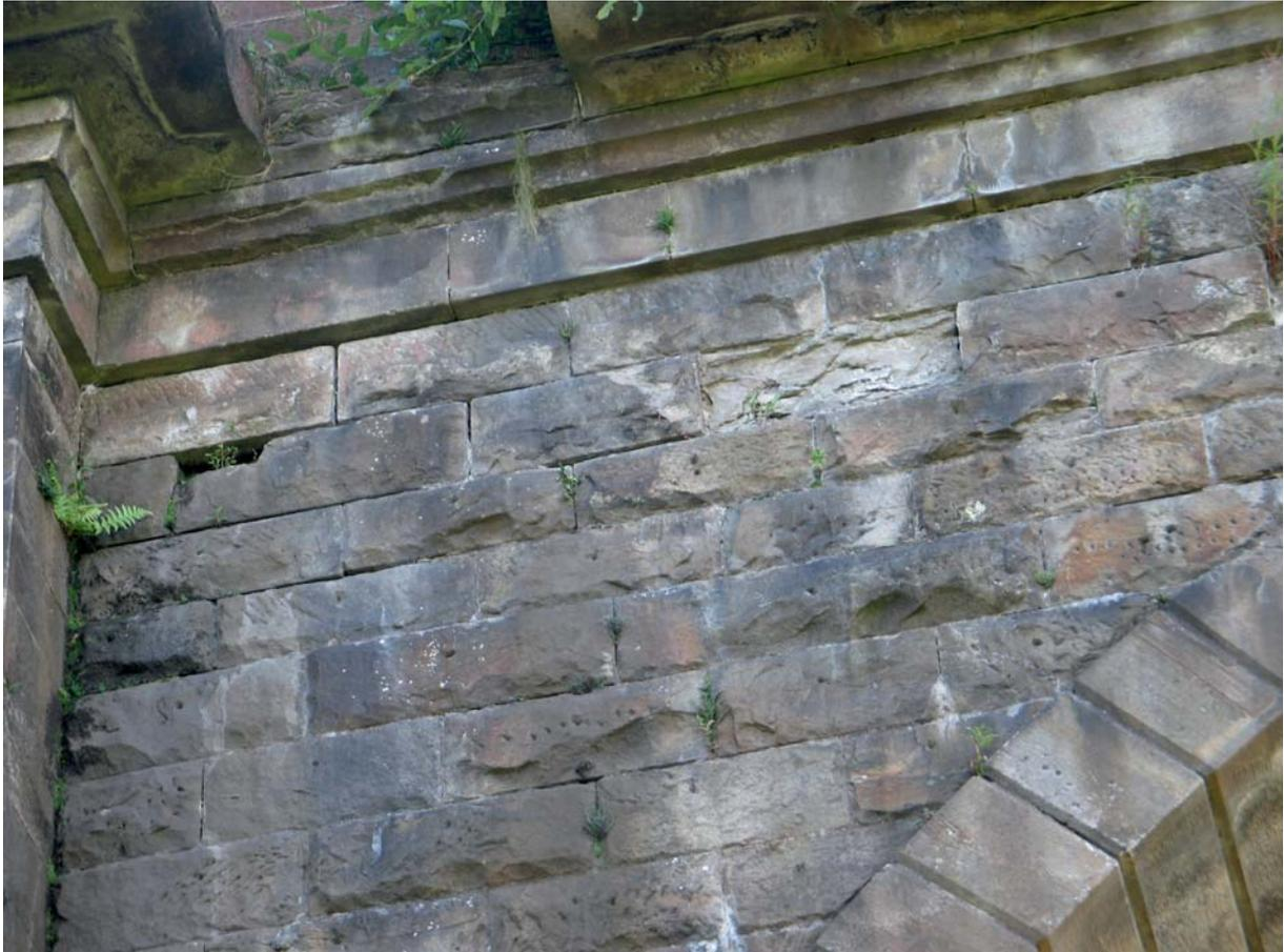
The stone was described by the masons as Freestone. In theory, that meant it could be cut and dressed in any direction but here we can see one stone which has been cut against the grain. Is that lack of skill on the part of the mason concerned, lack of care or even simply that when green the stone showed no real evidence of bedding?
