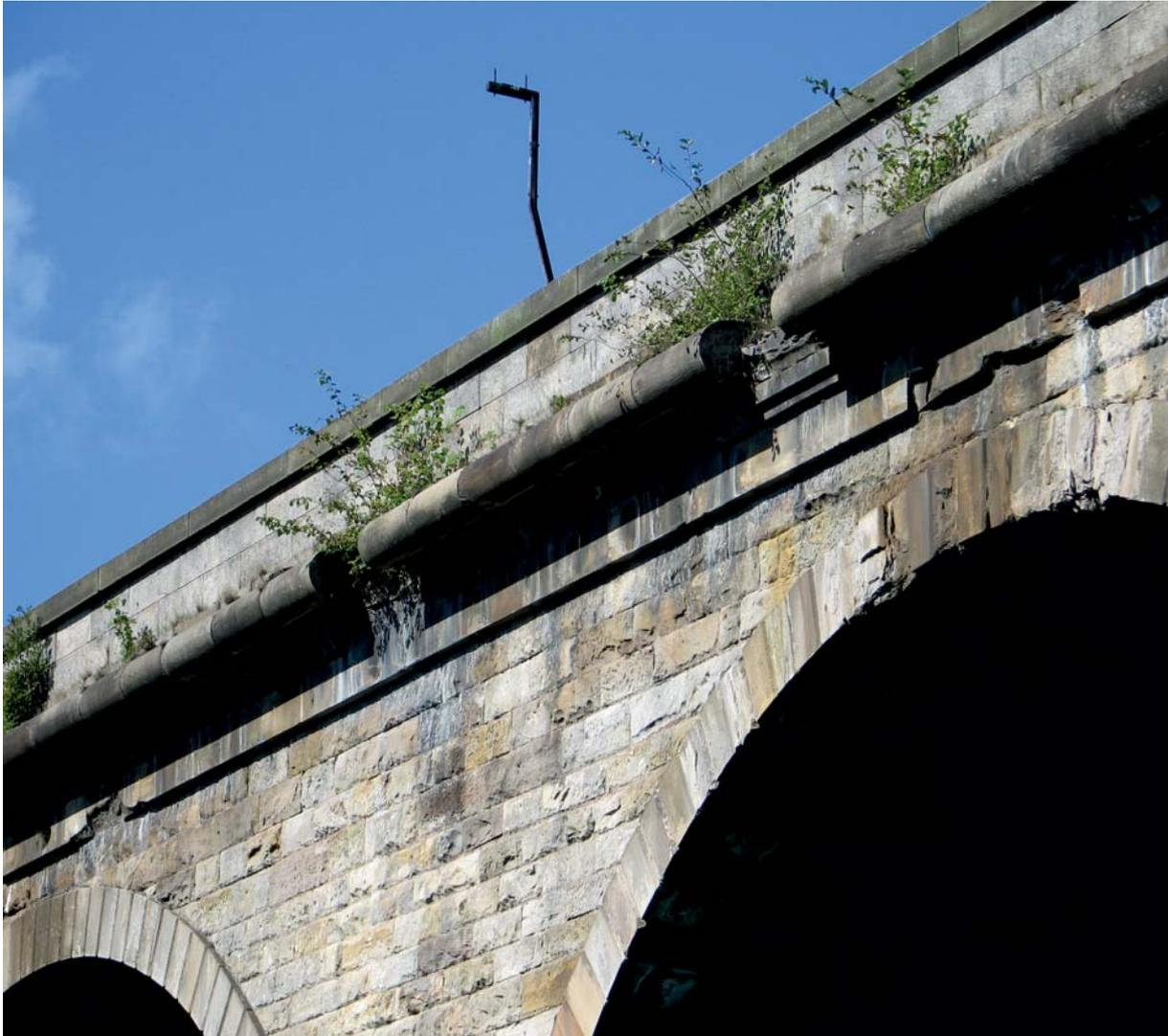
The scale of the stones used is clear from the nosings, some of which have broken off. The arch ring is about 30in thick and the nosings are only slightly smaller, perhaps 2ft thick, 3ft long and at least 3ft back into the wall to provide stability (see also the section on page 6).
