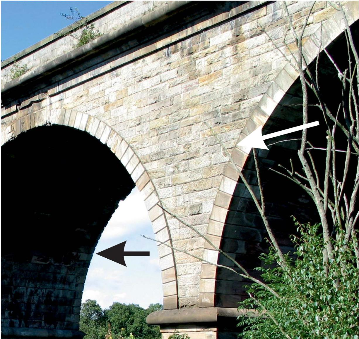
The arrows here mark the points where the construction changes. Both the spandrel wall and the arch soffit show different weathering above and below the line where the masonry is solid through. The upper level of the internal voids corresponds with the ashlar course below the (somewhat fractured) nose. Careful inspection of the first photograph will show that there are water runs on the surface of this ashlar which come from the top level of the deck slabs.
