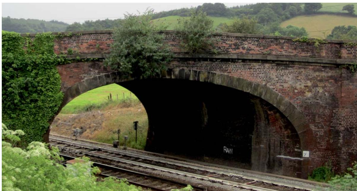
This is a skew bridge, and the first thing to note is that it presents an almost semi-elliptical form when viewed square to the spandrel. A track aligned view is, of course, not possible from accessible places but I am confident from the plotting I have done that the bridge is a semi circle on the square span.
