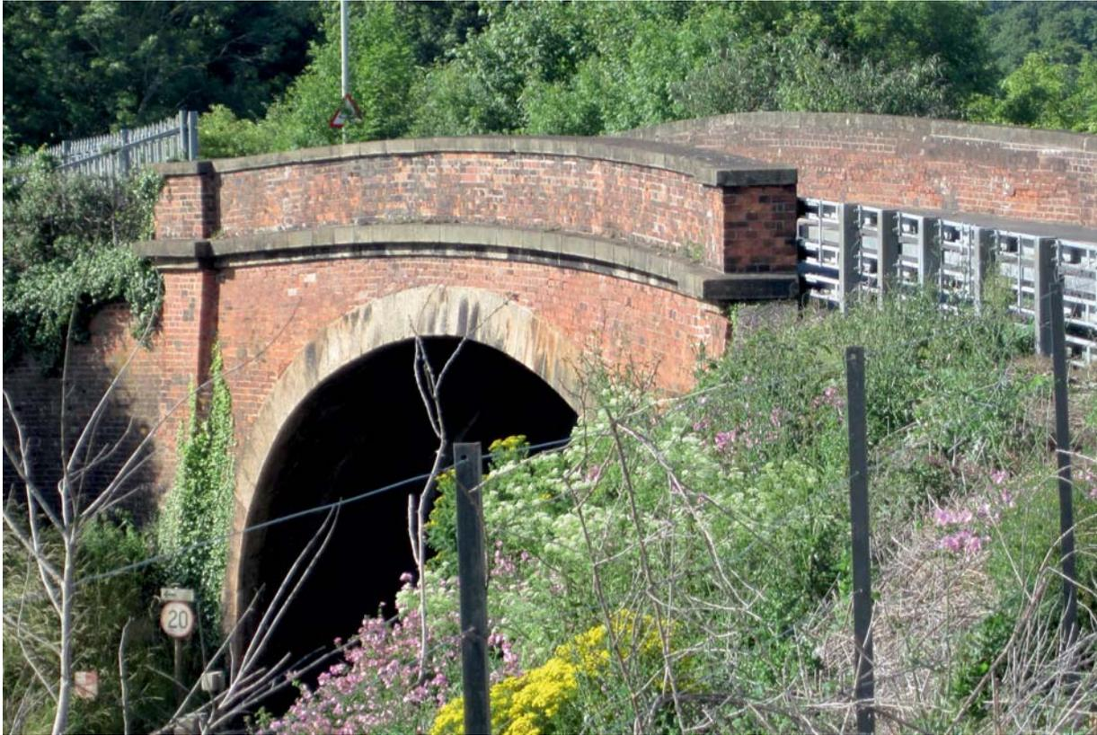
This view shows the curve and tilt of the spandrel wall. It is interesting to note that the string course, the coping and the brick courses of the parapet all follow the same curve. That must have been difficult to build.
