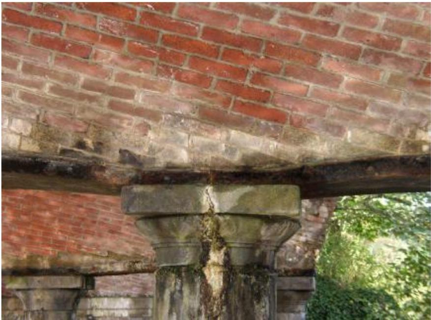
But none of that is the reason for showing this bridge. The important thing is what it has to teach us about skew arch behaviour. The established view is that skew bridges try to span square. Even if that is true, the centre of thrust at mid span must be at the centre of the bridge width. Drawing that effect shows that the resulting forces on the piers create a substantial moment in plan (below).
