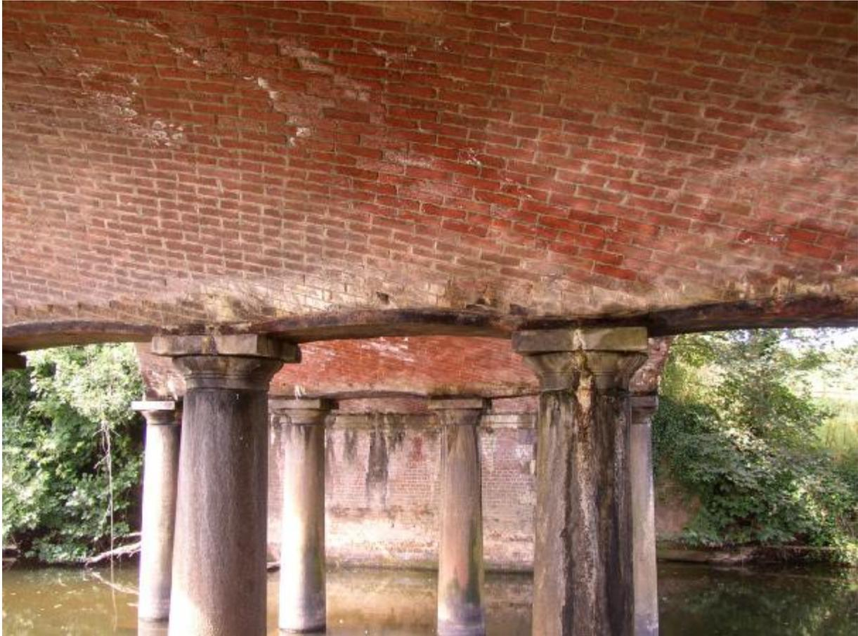
You can see, here, how the shoes divide in the middle of the piers. Any joints in the stone are well disguised. Indeed, it was only on closer examination of these photographs that I detected the illusion created by marking up brick shapes on the stone face. A closer look, below, shows how the cap stone of the pier column has split. It also shows the change from real to drawn bricks. That is even more visible on the further pier.
